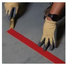
8. To remove Tough-Mark™ strips and shapes, starting at the edge, use a scraper to break the bond between the strip / shape and the floor. Once the edge is lifted peel back the tape to remove.
