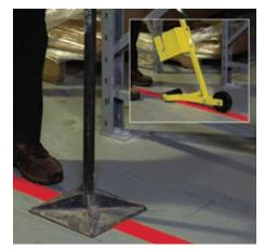
For maximum adhesion, use a tamper device with a minimum of a 150-pound load. Tamp in the same direction that the strips were applied. Several passes should ensure adhesion to the surface.
